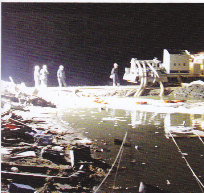
Pumping cars drain water at (l) Watari Town, Miyagi, Japan after the earthquake and tsunami in March 2011 and (r) Bangkadi Industrial Park, Bangkok, Thailand during the Chao Phraya flood in November 2011.
